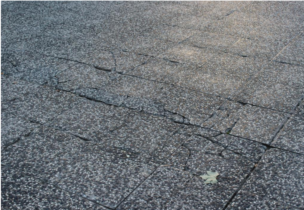
13. Tiles raised and in poor condition. It is agreed to keep the proposal: fix tiles
