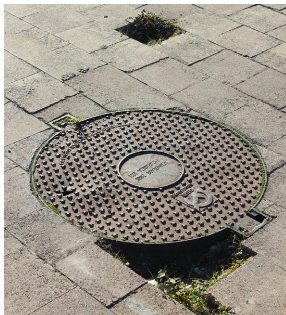
23. Holes and danger of tripping with tiles and sewer It is agreed to keep the proposal: fill and fix tiles and sewer
