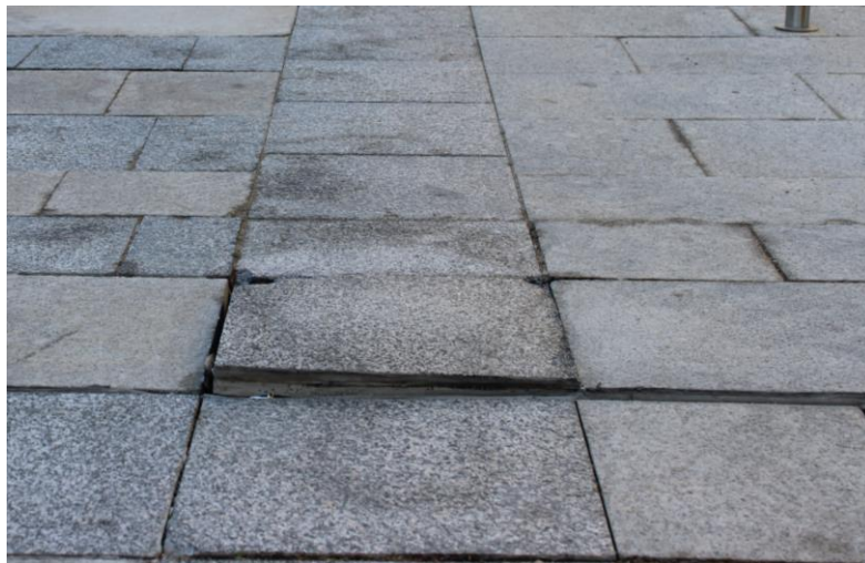
23. Holes and danger of tripping with tiles and sewer It is agreed to keep the proposal: fill and fix tiles and sewer
