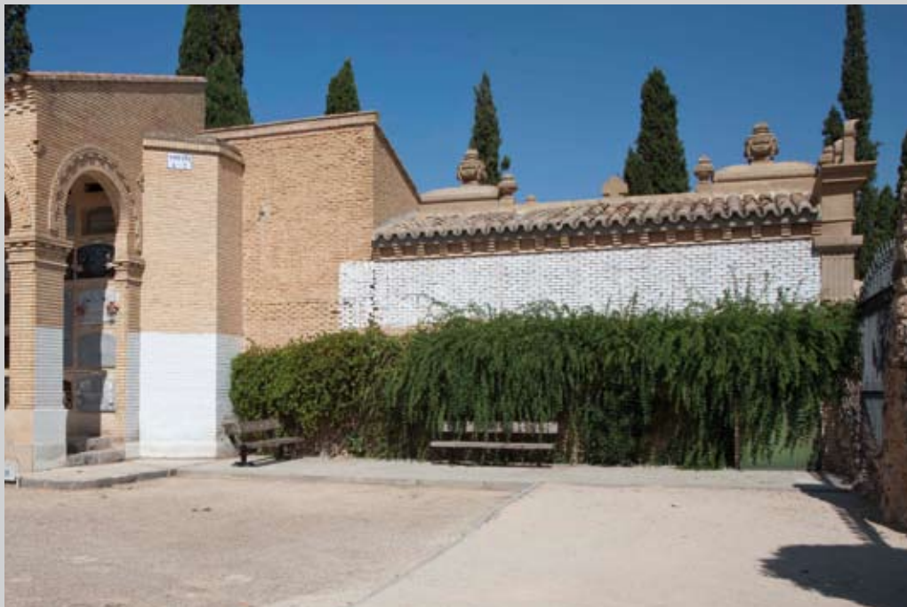
Execution site (back wall of the cemetery in 1936)
